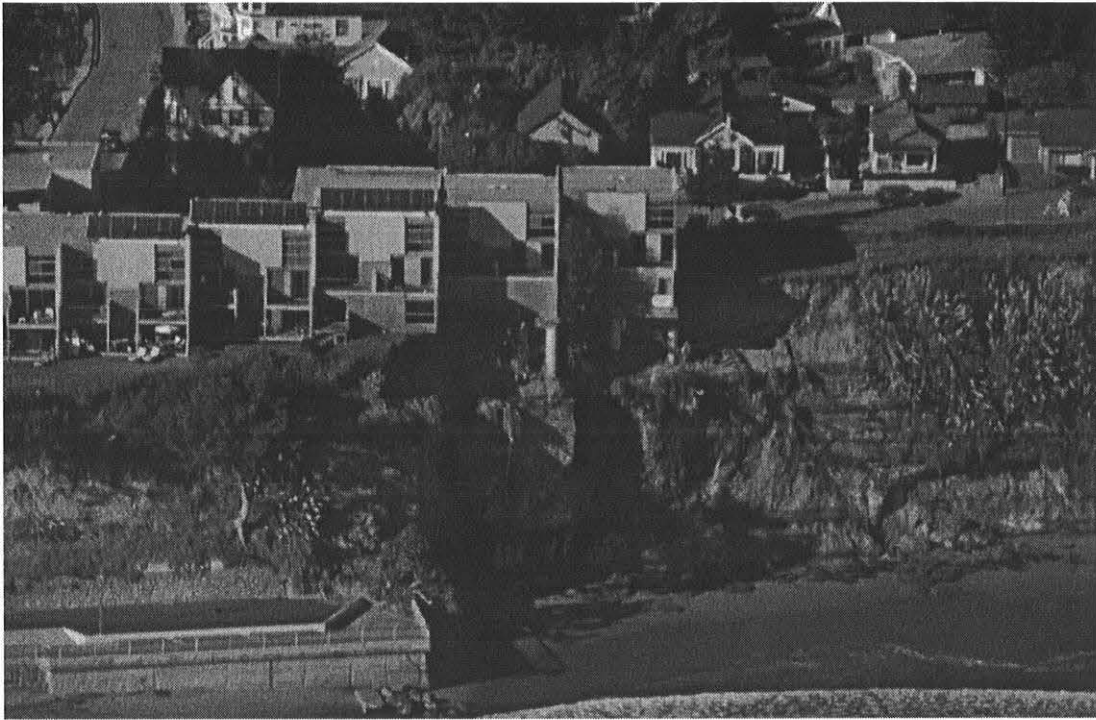
Figure 4a. An apartment complex overhanging the cliff edge in Capitola before the 1989 Loma Prieta earthquake.
