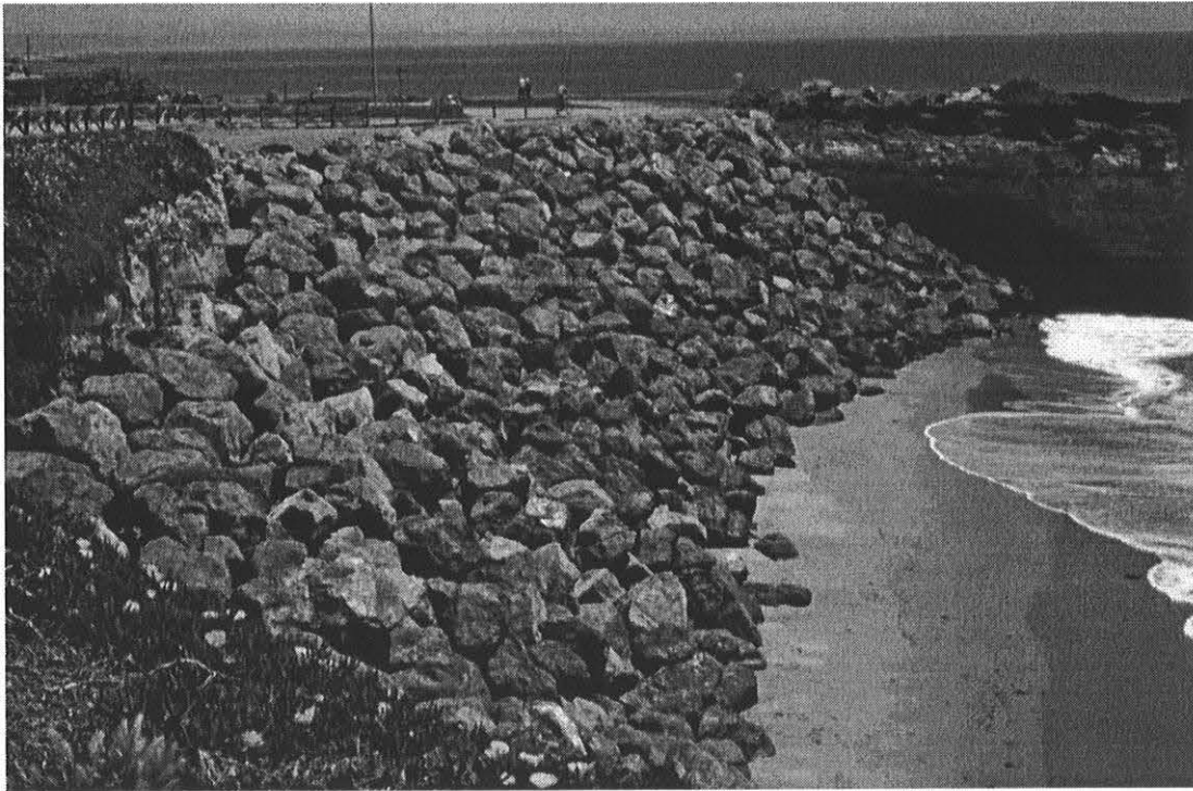
Figure 9. The placement of a large revetment will lead to the direct loss of much of the beach due to beach area taken up by the rock.
