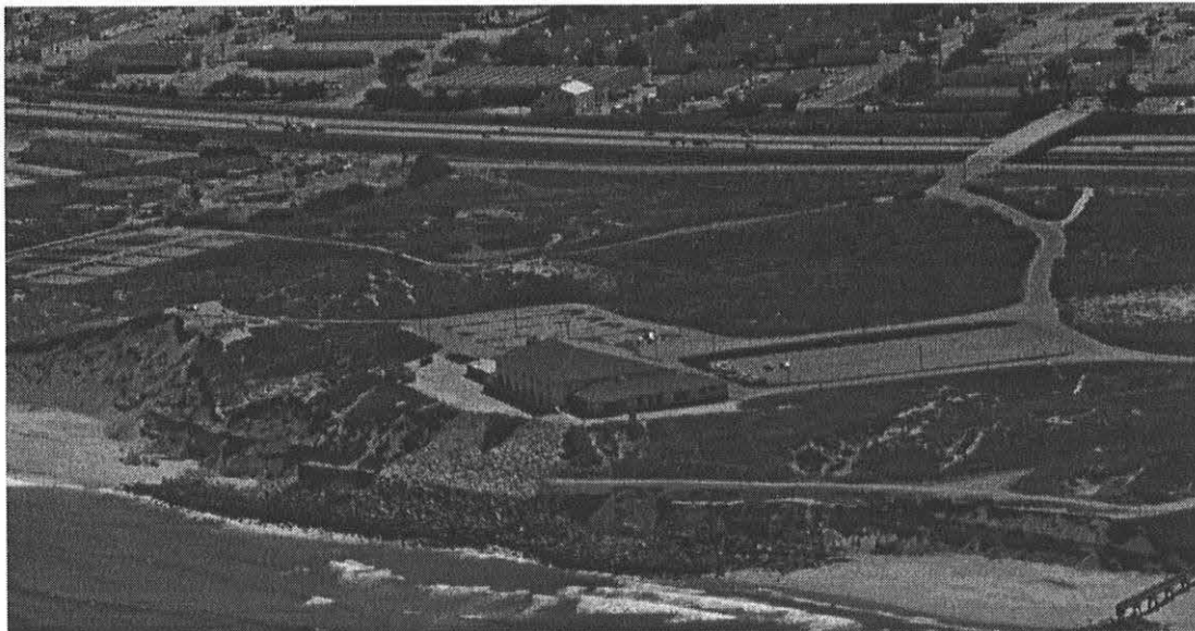
Figure 10. Passive erosion in the Ft. Ord area of central Monterey Bay. A beach still exists to either side of the rip-rap because the sandy bluffs have continued to erode. In front of the rip-rap, however, the beach has been lost due to passive erosion.
