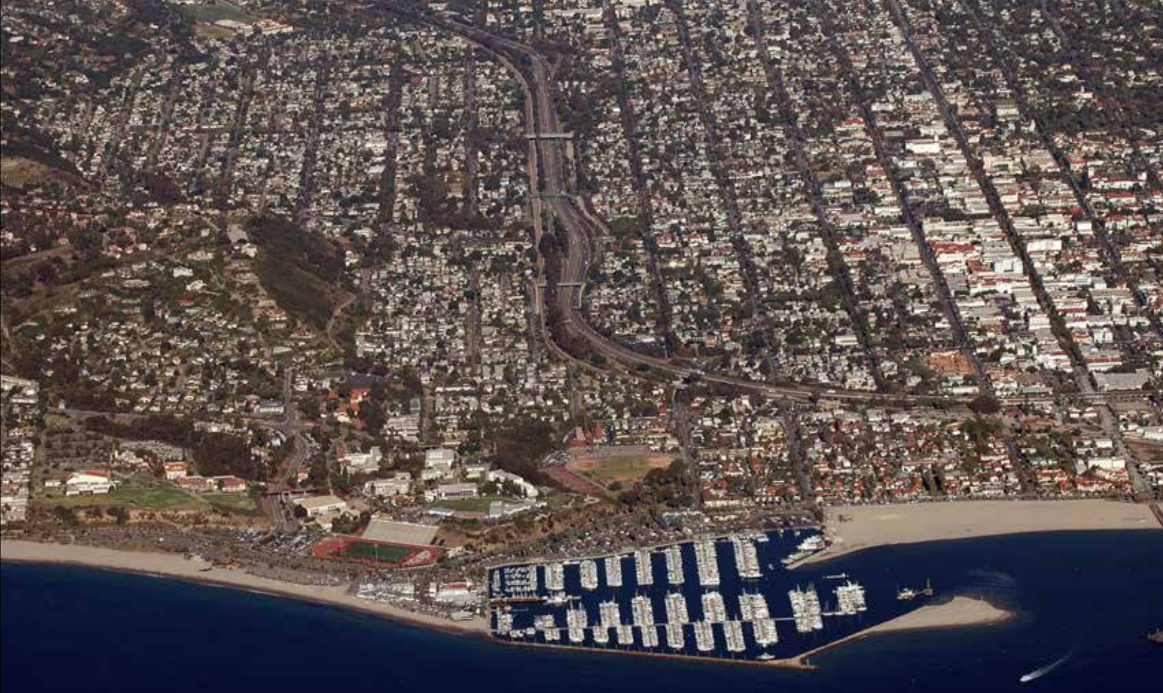
Figure 12. A breakwater at Santa Barbara trapped millions of cubic yards of sand following construction in 1928-1930 Courtesy: Bruce Perry, California State University Long Beach.
