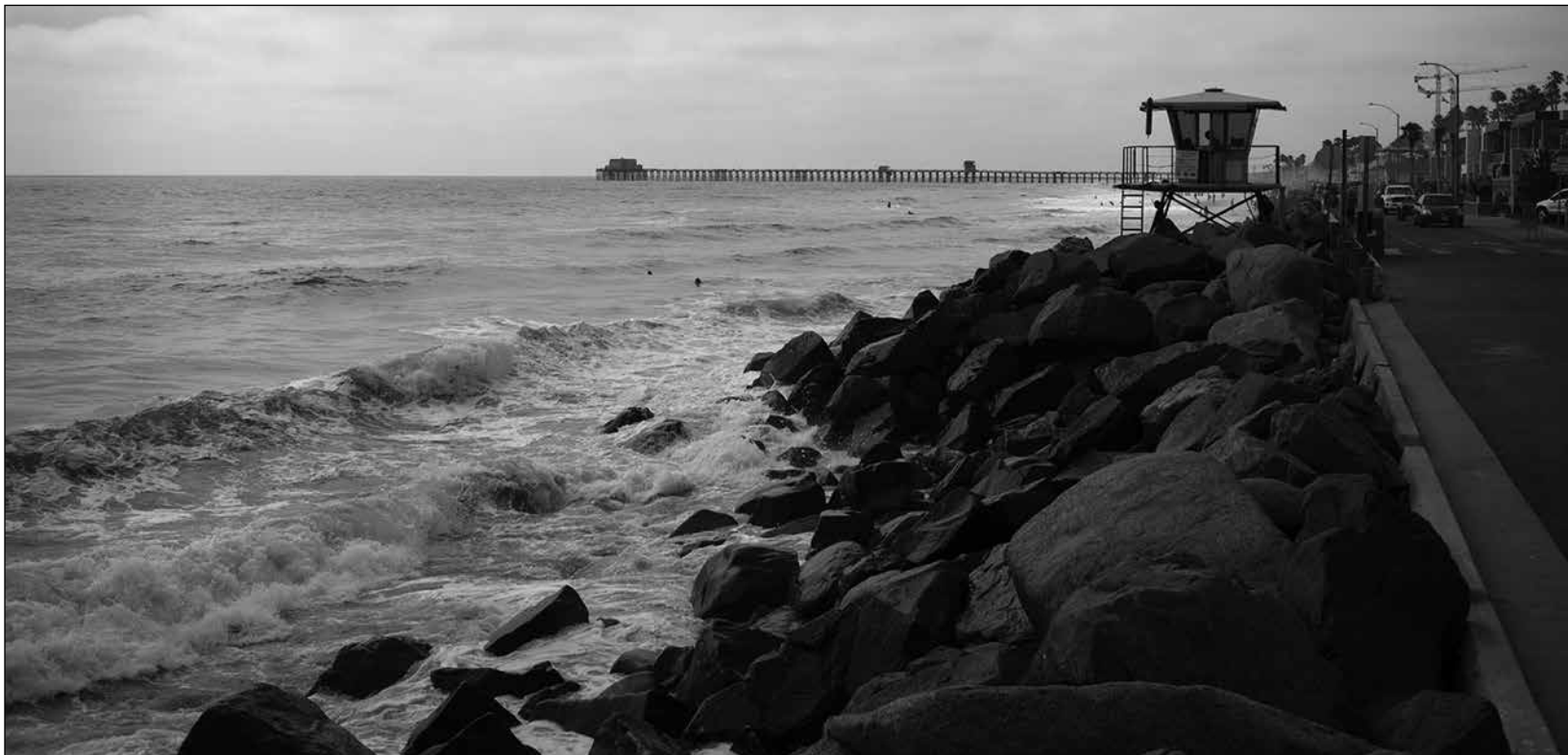
Figure 24. South Oceanside, showing riprap and narrow to nonexistent beaches. Image taken from just south of Wisconsin Street in July 2019. Photo: Ryan Anderson.
