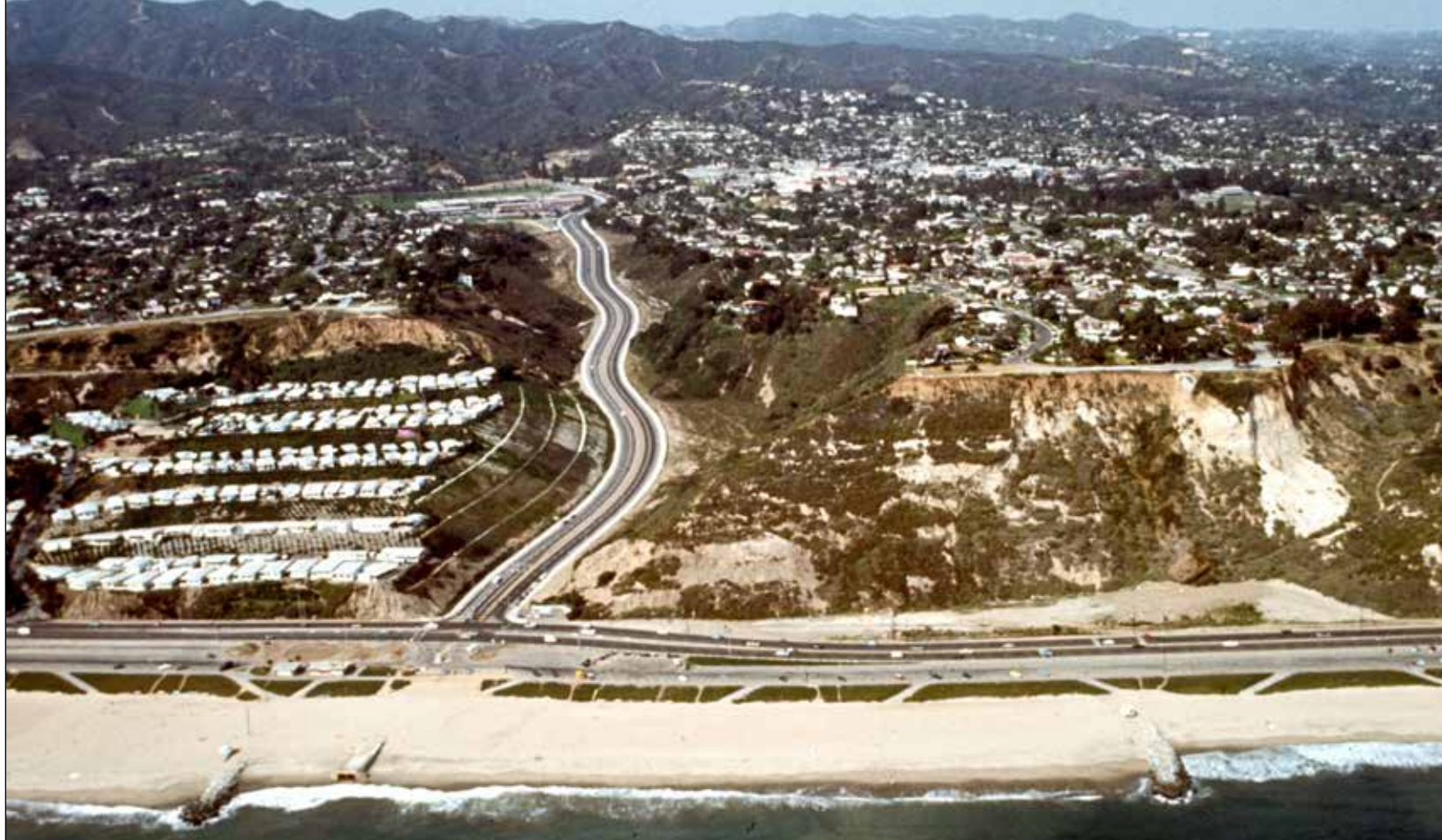
Figure 19. Groins at the northern end of Santa Monica shoreline in 1972. Courtesy: California Coastal Records Project.
