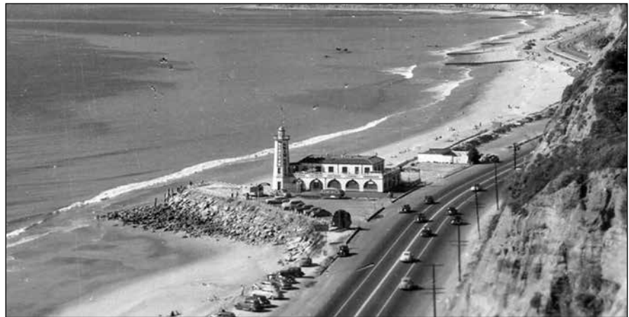
Figure 15. Original Las Tunas groin field along the eastern Malibu shoreline (in background).
