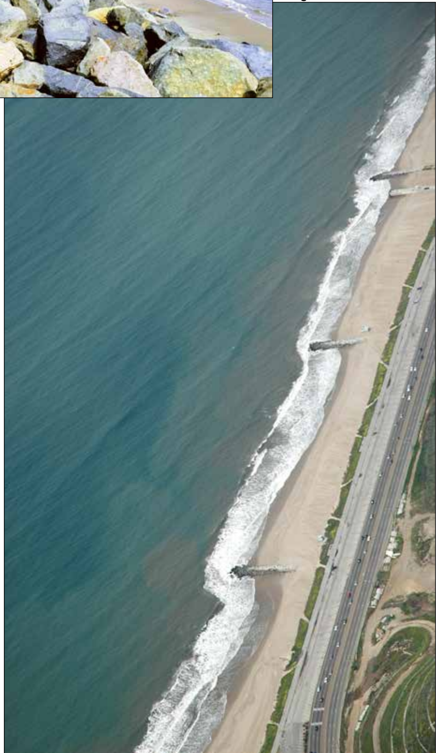
Figure 18 (below). Groins along the northern end of the Santa Monica shoreline. Courtesy: Bruce Perry, California State University Long Beach.
