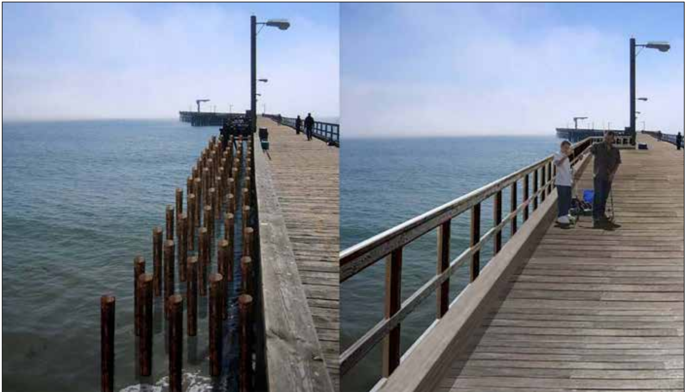
Figure 27. Visual simulation of proposed permeable groin at Goleta Pier/Beach (CCC 2009).
