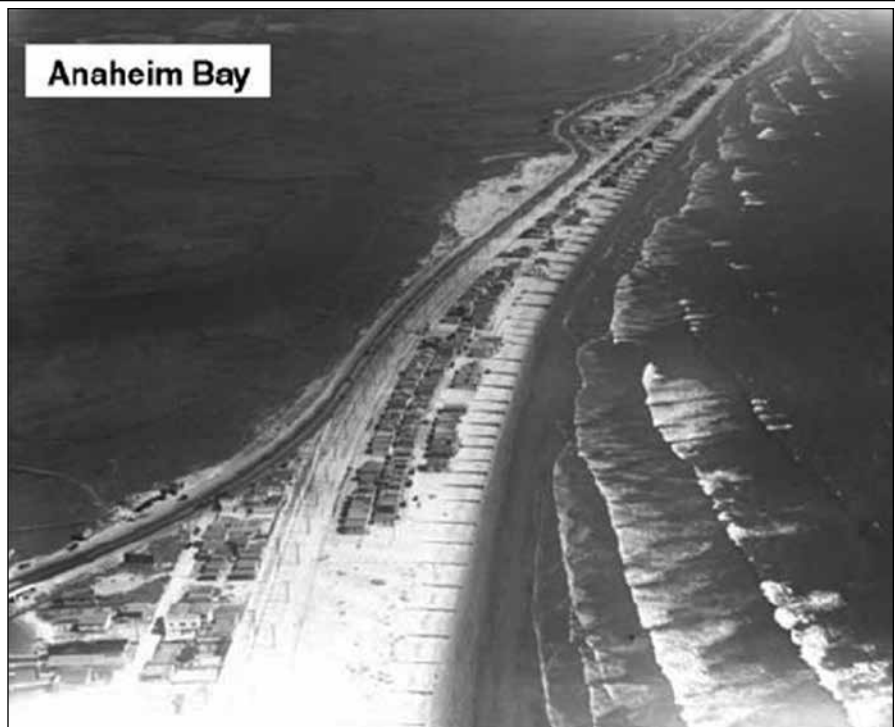
Figure 20. Residential development at Surfside in 1935, looking southward. The beach is very narrow and broken up by wooden groins. Spence Collections. Reproduced courtesy: Dept. of Geography, University of California Los Angeles.
