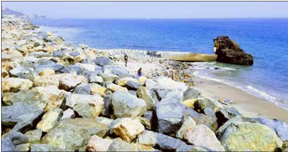
Figure 17 (left). Repaired groin, Las Tunas Beach, Los Angeles County, California. Photo: Kiki Patsch.
