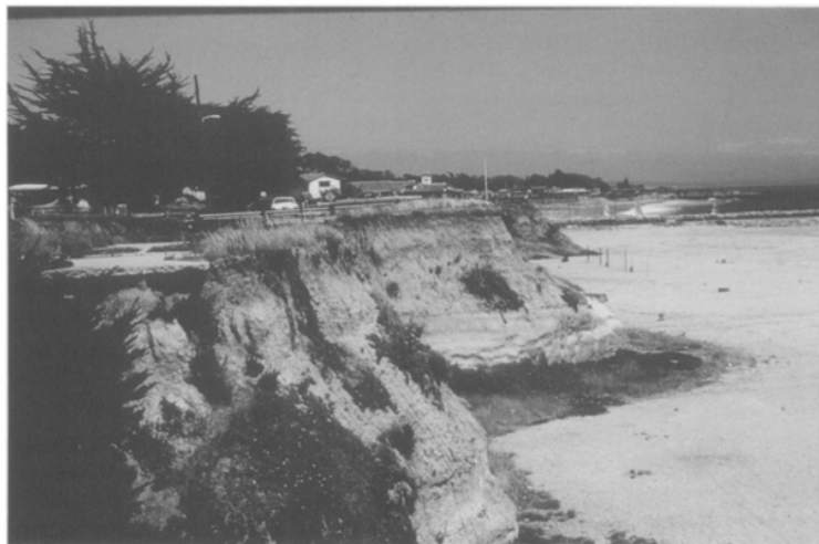
Figure 13. Remnants of the former ocean front street above Seabright Beach that was eroded prior to the construction of the harbor jetties at Santa Cruz. Note jetties in the background.
