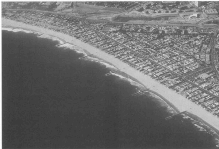
Figure 1. A groin field has been used effectively to stabilize and widen the beach at Ventura, California (1989).
