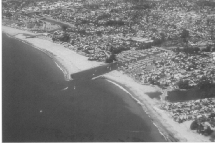
Figure 7. The jetties of the Santa Cruz small craft harbor and the upcoast beach (Seabright Beach) that has formed from trapping of littoral drift (1997).
