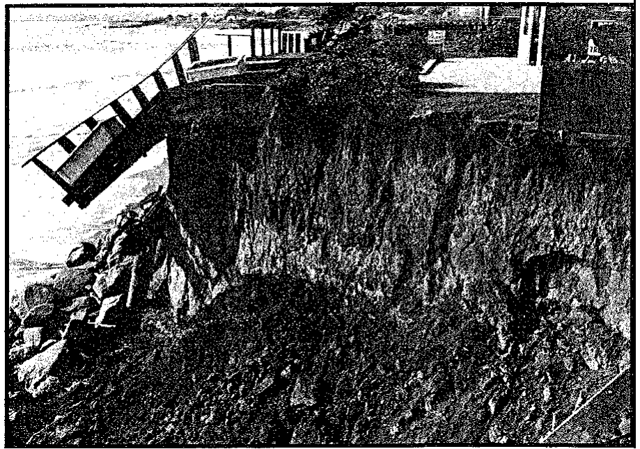
Photo 16. Rapid sea cliff retreat at the end of 26th Avenue in the East Cliff area of Santa Cruz. The lack of cliff protection at the end of a public road has led to lateral erosion of private property.
