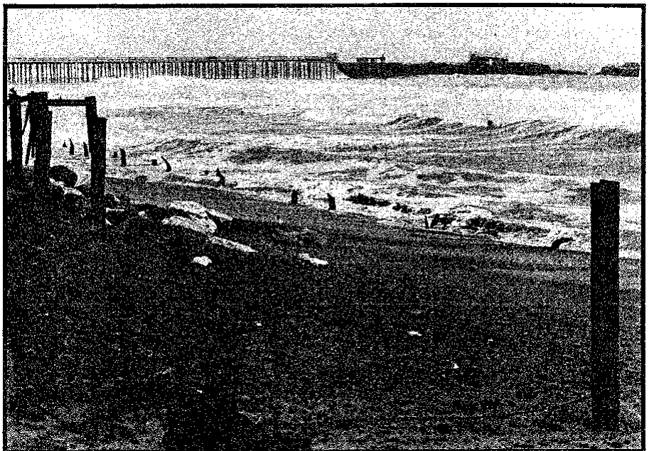
Photo 3. The remains of the Seacliff seawall in March 1983. Approximately 240 meters of a new 800 meter long piling and timber bulkhead were totally destroyed during January 1983 within 2 months of completion.
