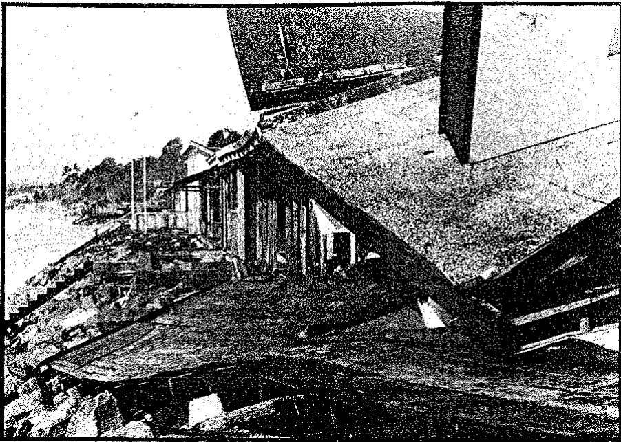
Photo 12. The roof of this ocean front house at Aptos Seascapes collapsed when waves destroyed the front wall in January 1983.
