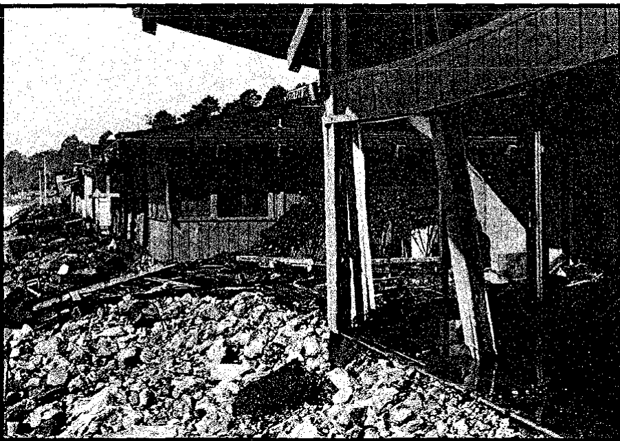
Photo 11. Wave damage to house fronts at Aptos Seascape. Waves created major structural damage by removing supporting posts and walls.
