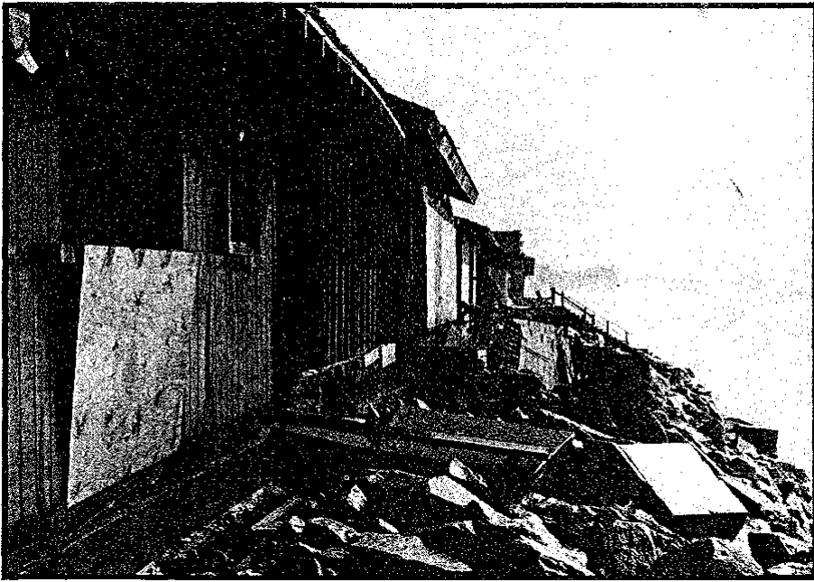
Photo 10. Wave damage to ocean front homes at Aptos Seascape during January 1983. Although these homes were elevated 3-4 meters above the beach and partially protected by a rip-rap seawall, wave overtopping led to damage to 19 of the 21 homes.
