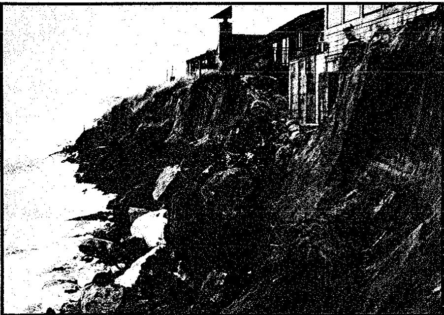
Photo 13. Erosion of dunes at Pajaro Dunes development in January 1983 exposed the foundations and threatened a number of homes. Rip-rap was brought in for emergency repair.
