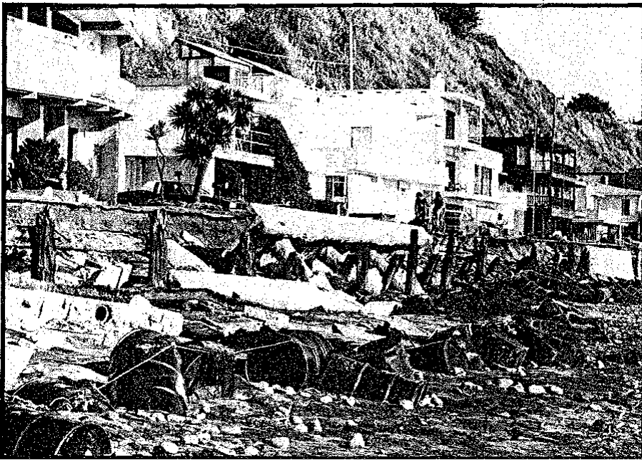
Photo 4. Storm damage during 1978 storms along Beach Drive in Rio Del Mar. Note remains of timber bulkhead and collapsed sidewalk. A temporary barrier of cabled oil drums failed almost immediately.
