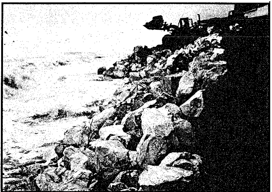
Photo 15. Emergency rip-rap was emplaced along almost a mile of ocean front at Pajaro Dunes during January 1983 storms.
