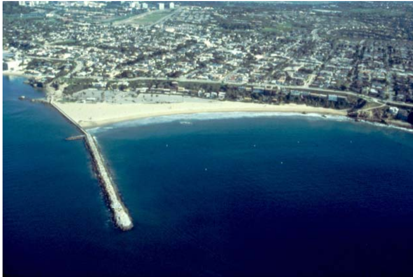
Figure 65. Big Corona Beach retained by a natural headland and the east jetty at the entrance to Newport Bay.
