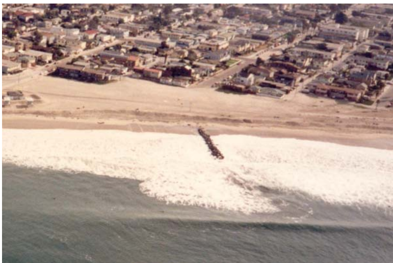
Figure 76. Ineffective groin at Ocean Beach, San Diego.
