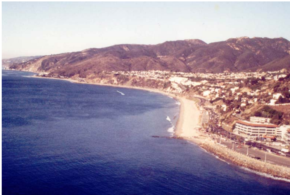
Figure 1. Fillet beach upcoast of a groin where Sunset Boulevard ends at the Pacific Ocean (near Santa Monica).
