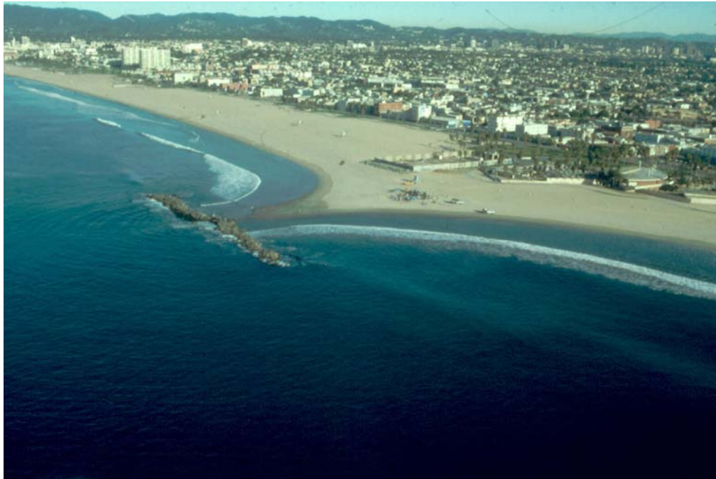
Figure 2. Salient in the lee of a detached breakwater at Venice.
