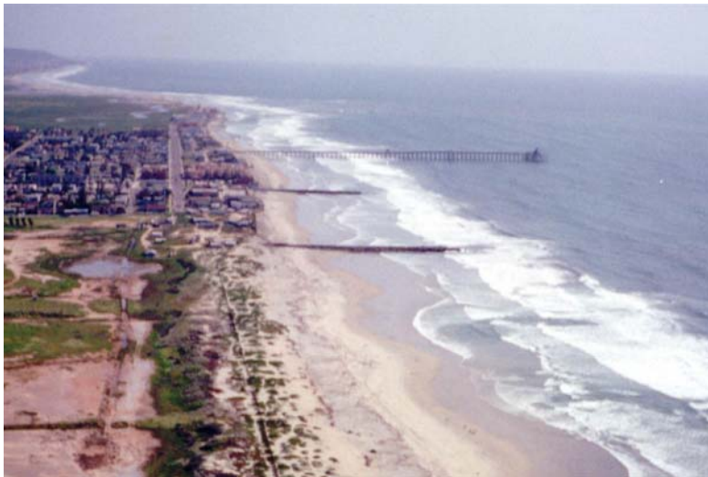
Figure 75. Lack of a fillet beach on either side of groins at Imperial Beach.
