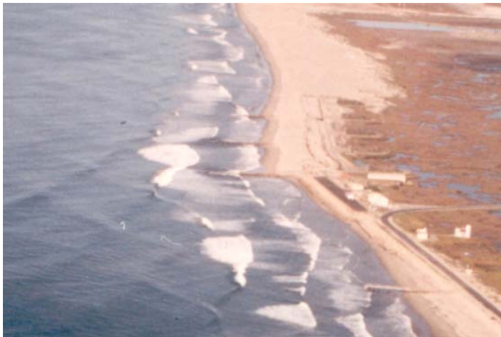
Figure 28. US Navy groins downcoast of Port Hueneme (1992 photo).
