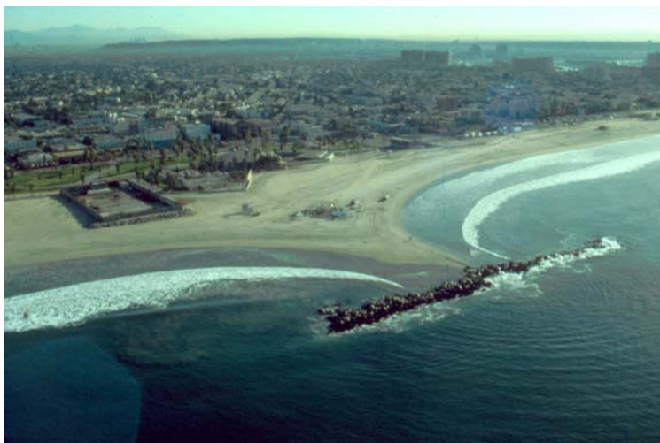
Figure 33. Venice salient and breakwater: note the groin that retains sand mostly on its upcoast side.
