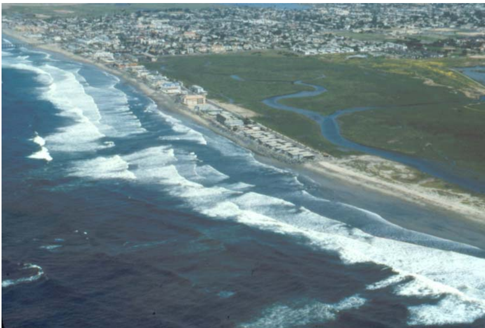
Figure 49. Revetment protecting homes on the sand spit in the lee of the rocky delta of the Tijuana River at Imperial Beach.
