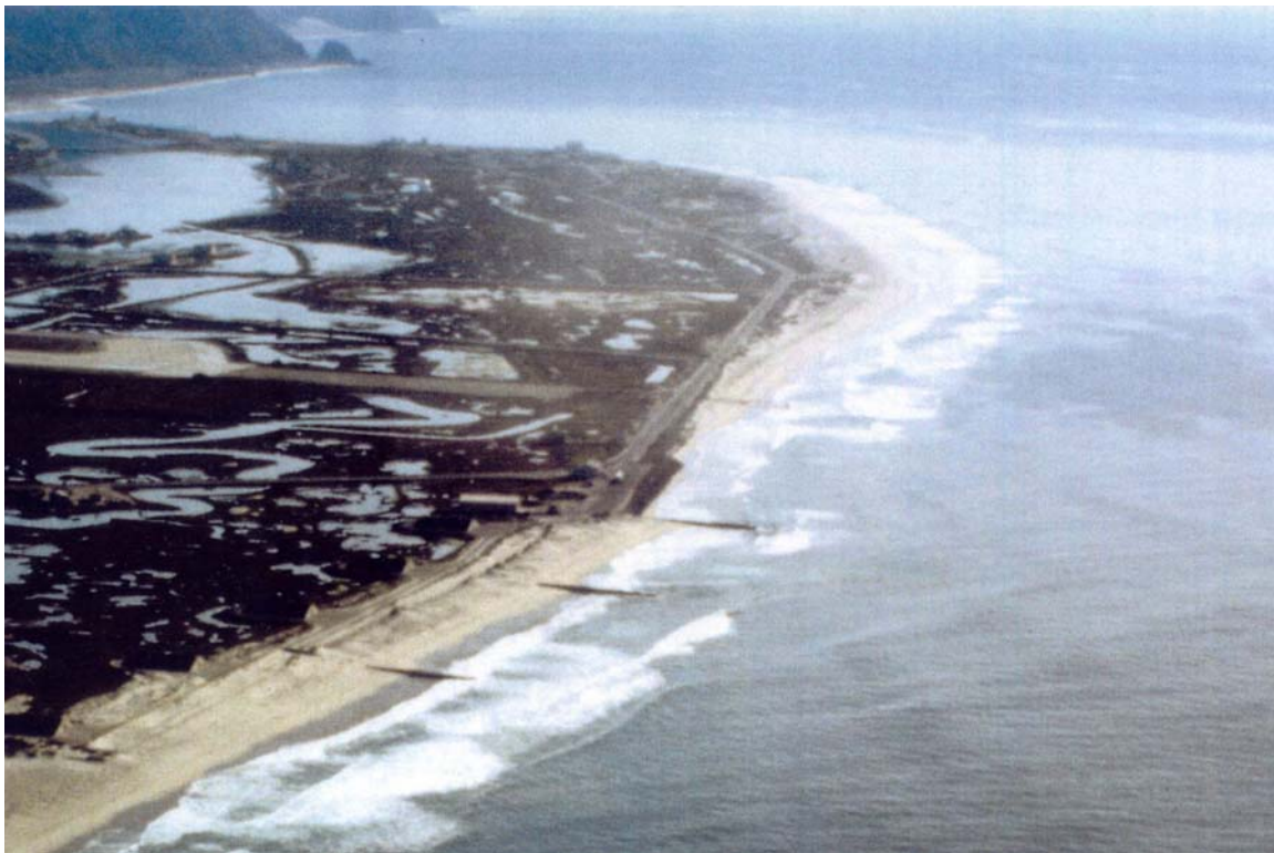
Figure 30. Revetment downcoast of the east or last groin along the US Navy coast between Hueneme Beach and Point Mugu; Laguna Point at upper right (1992 photo).
