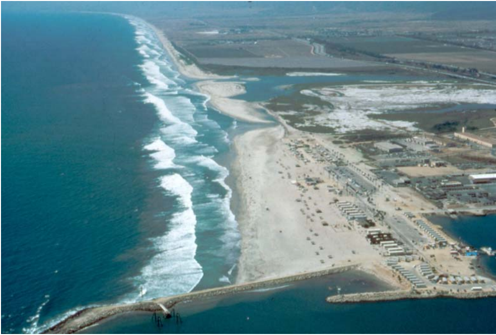
Figure 9. Shore-connected breakwater and the upcoast fillet beach at the north side of Oceanside Harbor (1990's photo).
