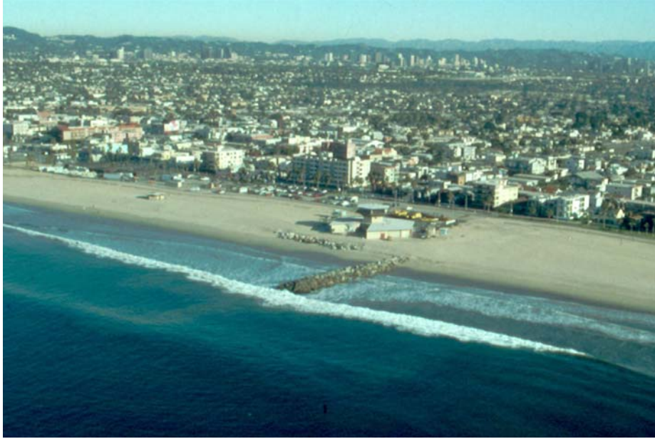
Figure 77. Ineffective groin at Venice, Los Angeles County.
