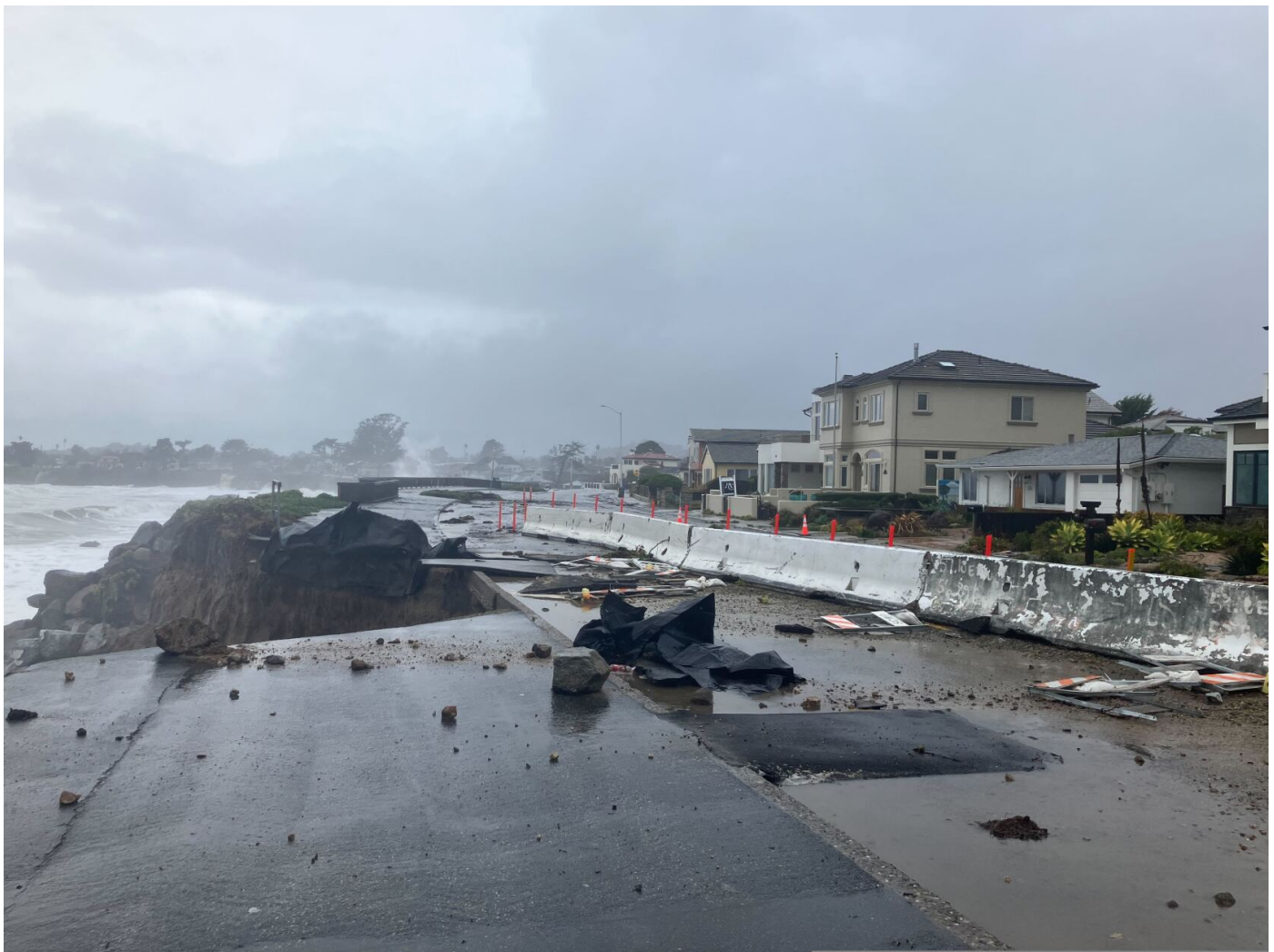
Storm surge in January severely damaged portions of West Cliff Drive in Santa Cruz.
